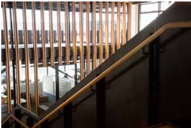
American White Oak stair and balustrade
